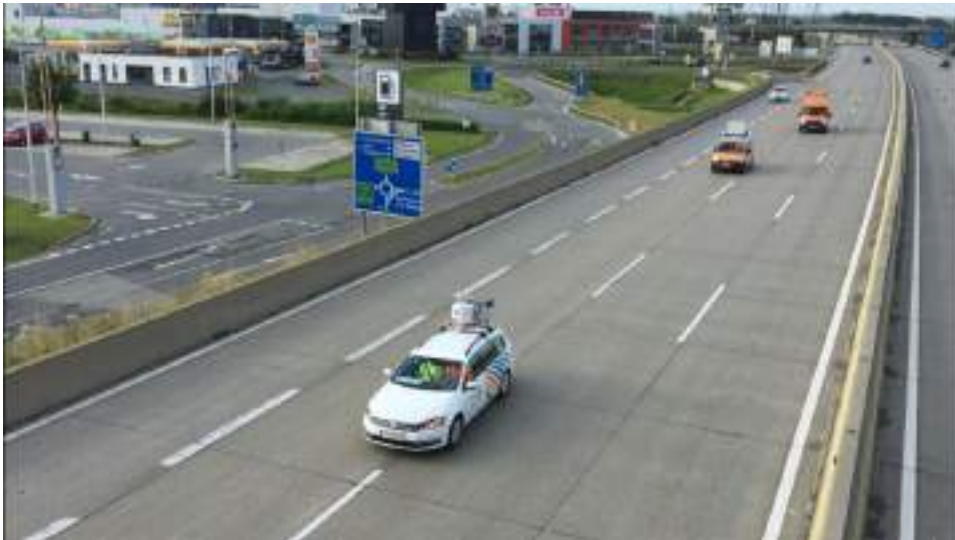
Public roads, Austrian highway A9
